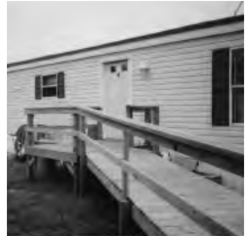
The Housing Advocacy and Assistance Program builds home access ramps, such as the one above, for Oswego County residents.
