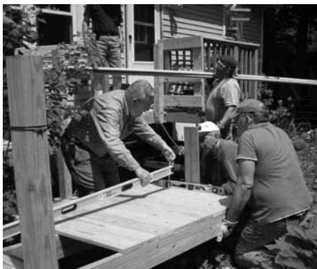
Volunteers at work building ramps.
